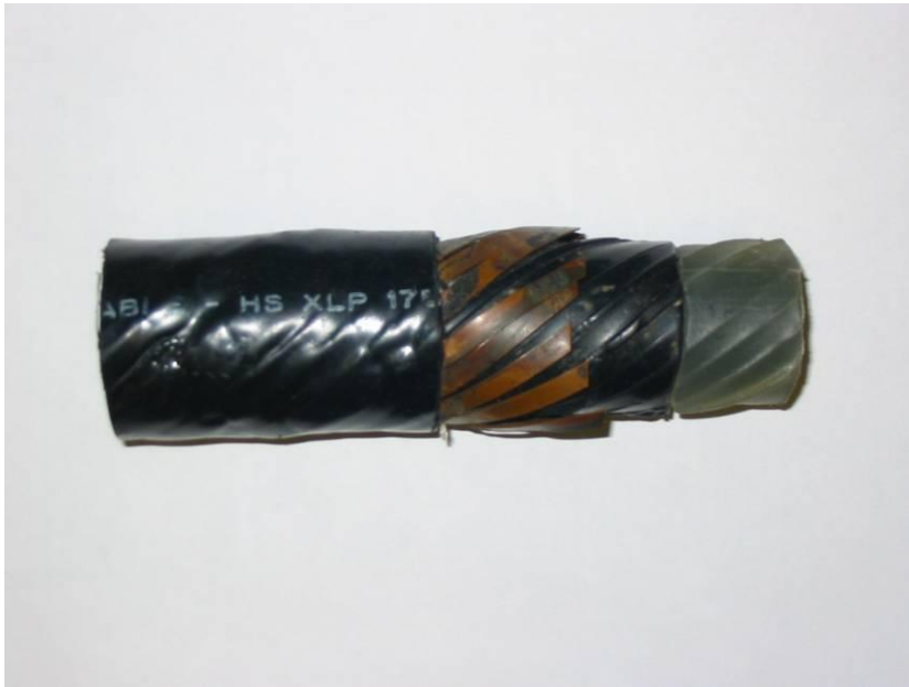
Overloading (Overheating) (Causes cable deformation)
