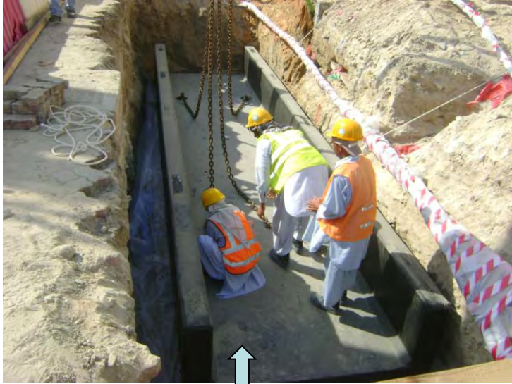
Joint Pit Installation
